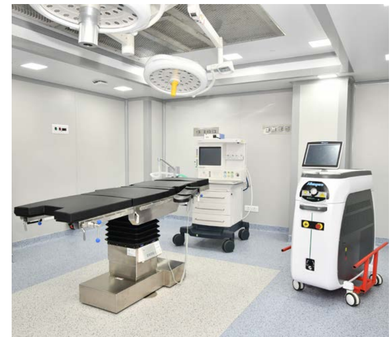
Renovated Gynecology Operation Theatre
